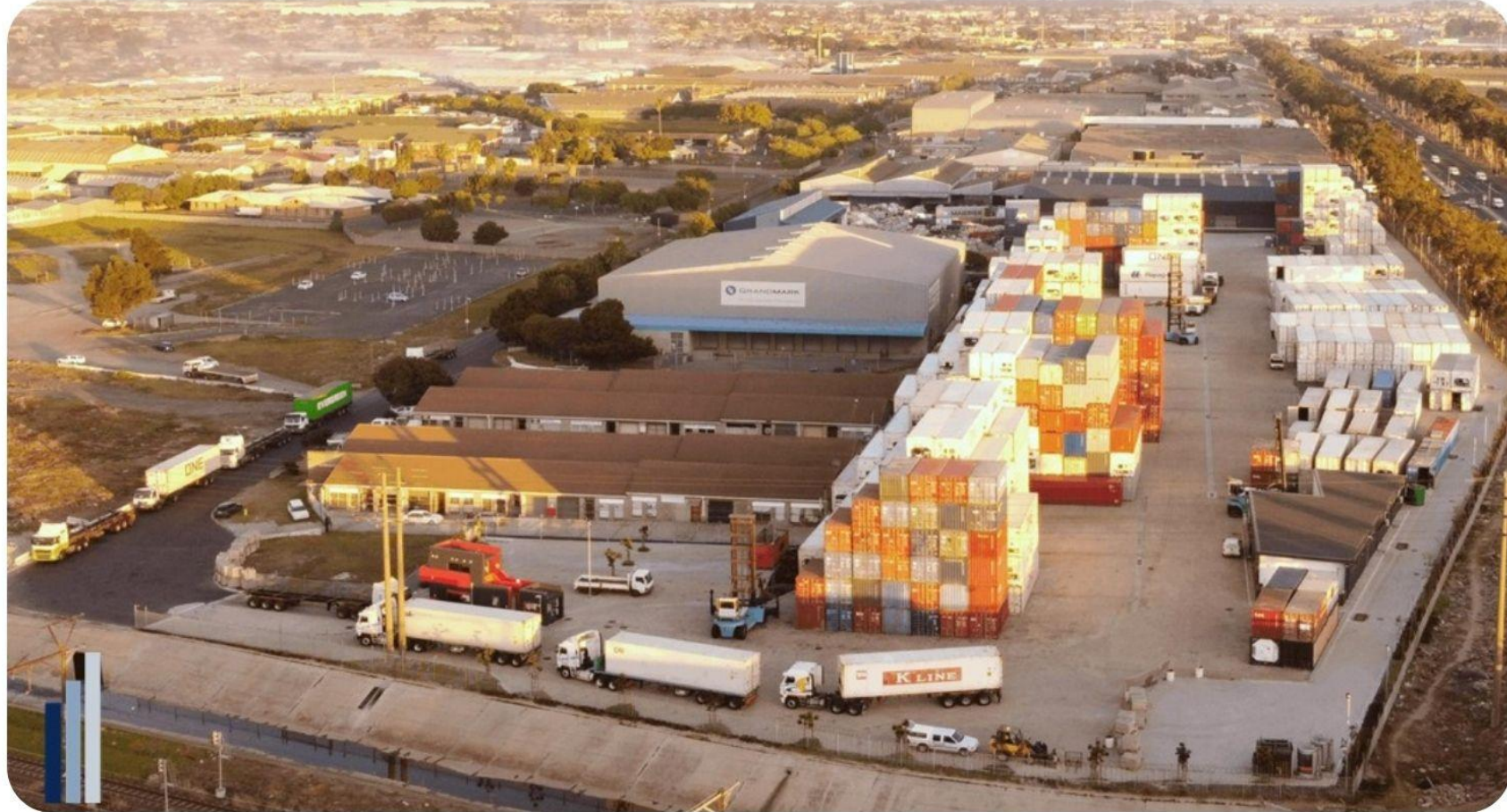
1 JAN SMUTS ROAD PAROW
